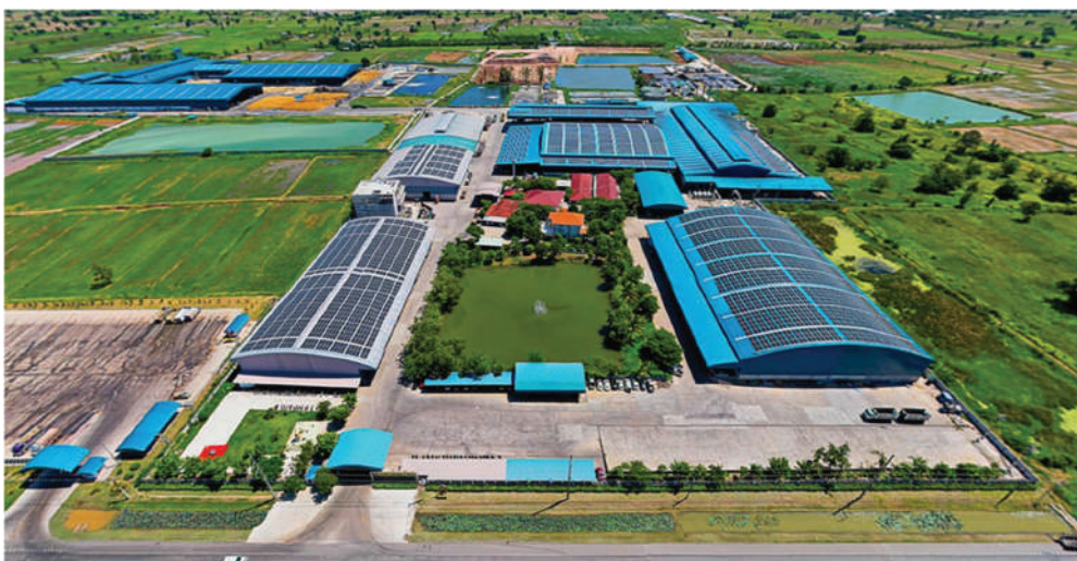
Rooftop solar panel power generation project
