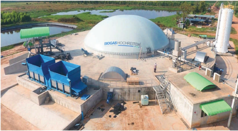
Napier grass biogas power generation project
